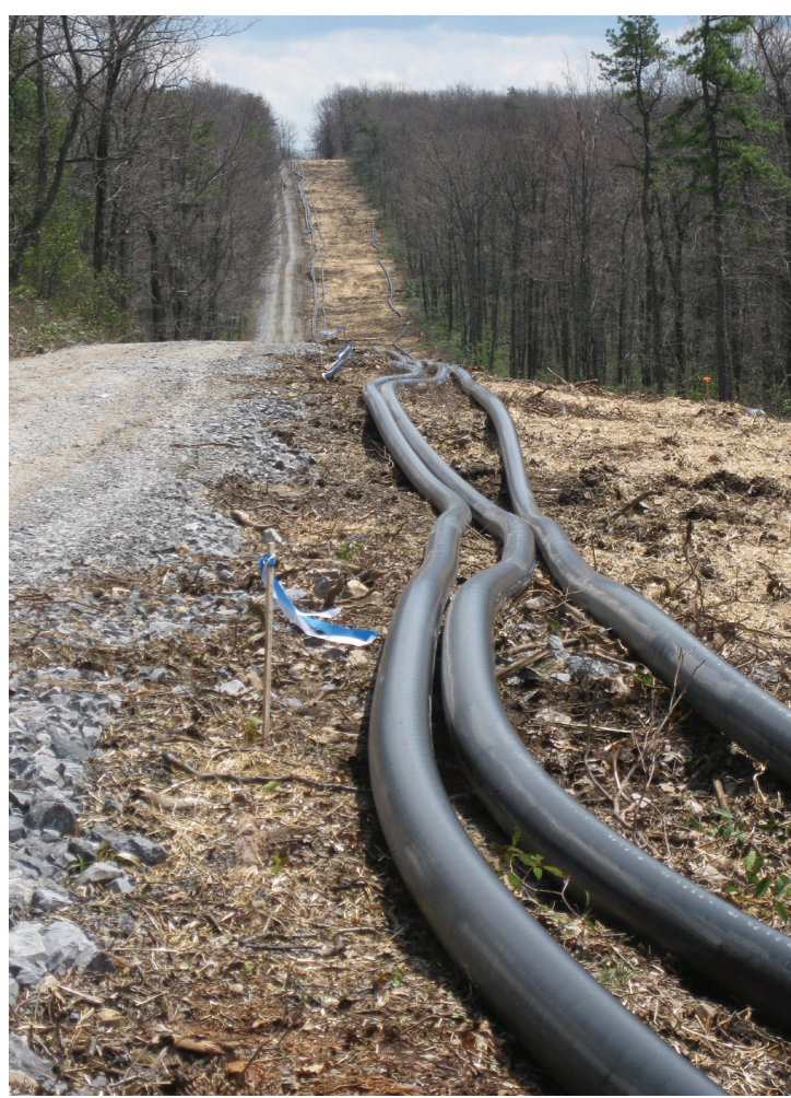
Anadarko's gas and water lines being laid on top of the mountain with the original dirt road being widened to accommodate them.
