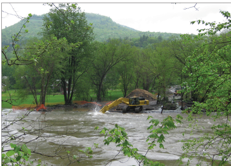
High water from recent rains washed away the coffer dam on Pine Creek! Lord knows how DEP, EPA, SRBC and PA Fish and Boat Commission will respond.
