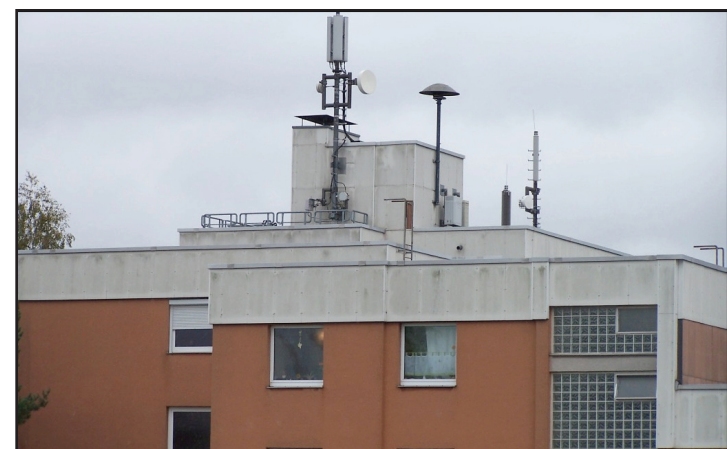
Cell Phone Transmitters on Top of the Multistory building at Feldstraße 28, Selbitz, Upper Franconia, Bavaria, Germany.
