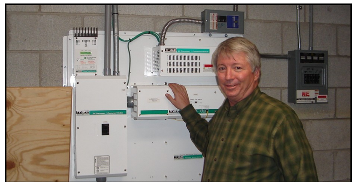
Fr. Charles points out the controls in the basement of the rectory for the solar panels on the roof. Morris, 57, was named to Rolling Stone magazine's Honor Roll last year for being a "man of his word" and leading other congregations to improve their energy efficiency.
