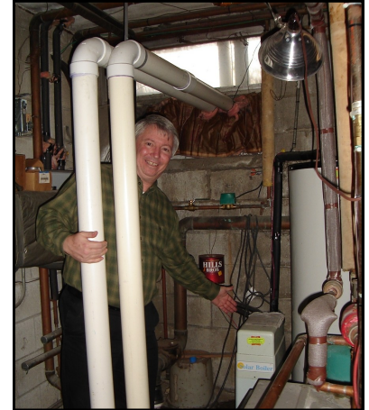
Rev. Charles Morris shows off pipes in the rectory basement that deliver water heated by the sun. The church saves about $20,000 a year on utility bills thanks to $150,000 worth of energy-saving investments the parish has made in the last few years.
