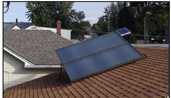
A solar fan on the rectory roof removes hot air from the attic, and another solar collector on the garage roof powers the pump which moves antifreeze through the solar water heater.
