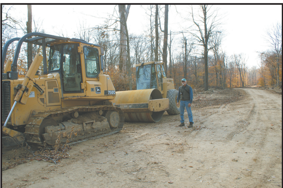
Bill Belitskus, founder of Friends of Rimrock, stands in front of equipment used to build a new road in Allegheny National Forest so that oil trucks and drilling equipment will have easy access to extract more fossil fuels from the ground. Photo by Terry Darling.
